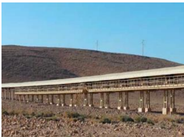
Cable belt conveyors
